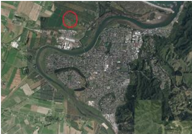
Figure 29: Keepa Rd, Green Waste Composting Facility
